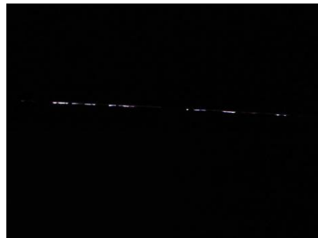
Side by side roof/wall joint with visible daylight at joint
