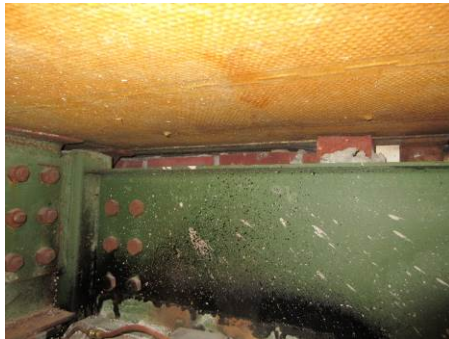
Side by side roof/wall joint with visible daylight at joint
