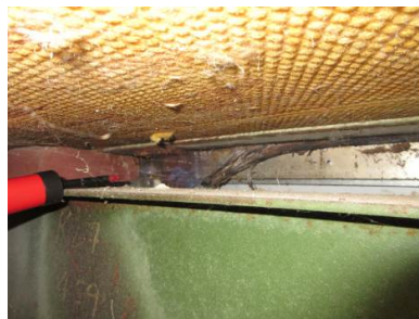
Roof/wall joint leakage diagnosed with Air-Current Tester
