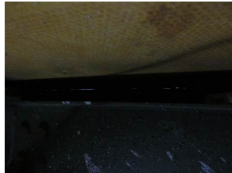
Side by side roof/wall joint with visible daylight at joint
