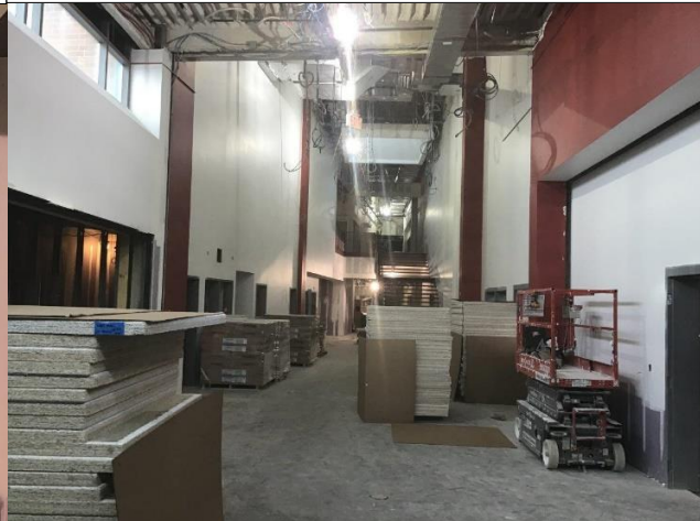
Main Lobby Looking At Stair 2
