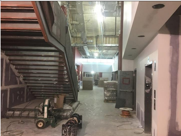
Main Lobby From Below Stair 2
