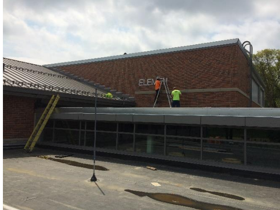
New Building Sign Installation
